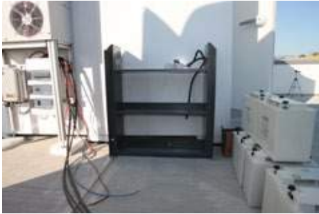
Installing the battery rack; on the left: chilling unit
