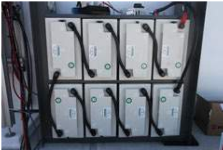
8 batteries make sure that the chilling unit will work 24/7
